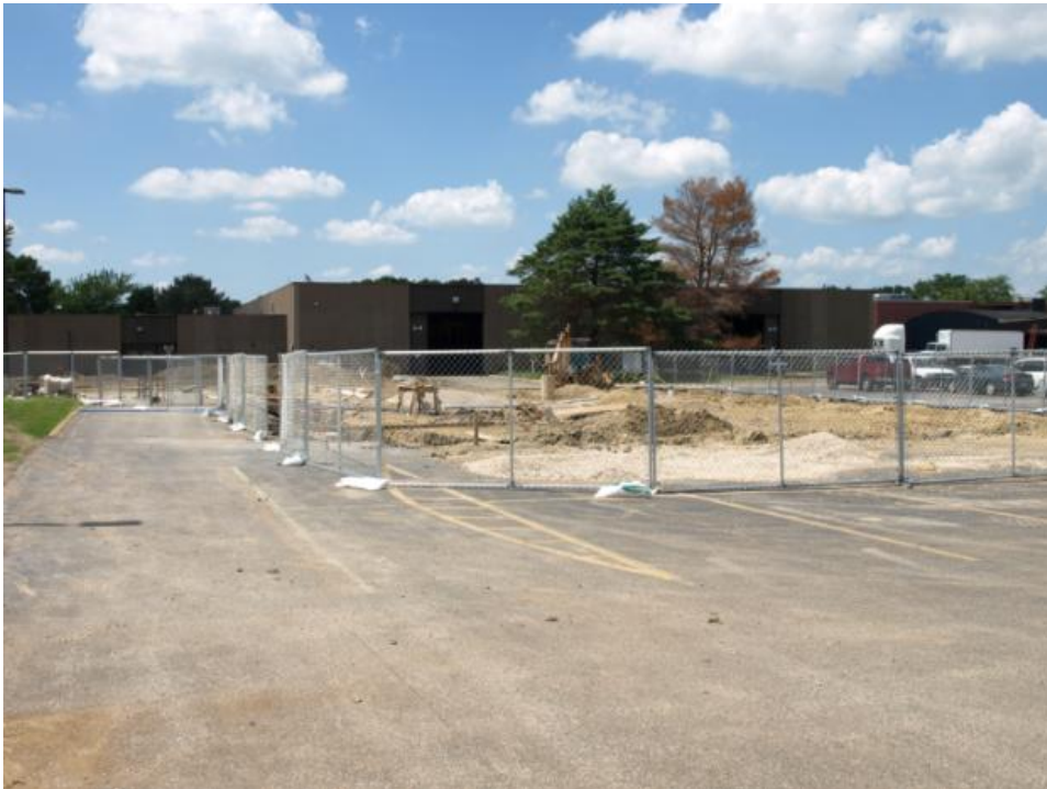
SCC Applied Technology Addition/Renovation Project
