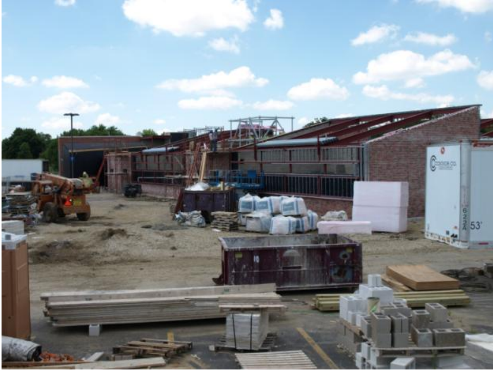
SCC Science Addition
